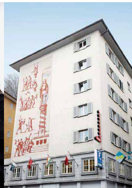
Student Residence, Baselstrasse
